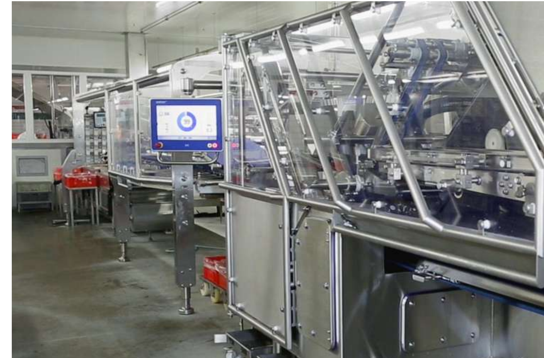
Machine line with new touch panel
